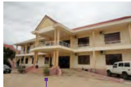
This is the Kampong Speu Provincial Health Department office. The training was held on the second floor of the building.
